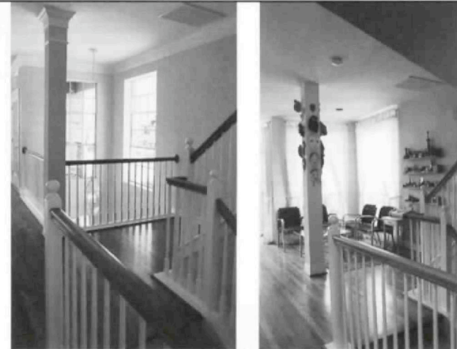
Before: A light well goes through from the second to the first floor. After: Closed in, the light well became a light-drenched seating nook.
