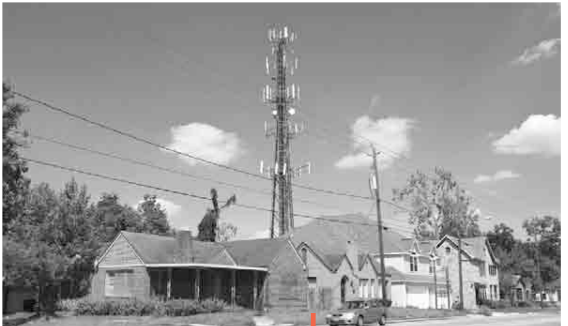
CELL PHONE TOWER, ALABAMA STREET BETWEEN HUTCHINS AND BASTROP STREETS.
