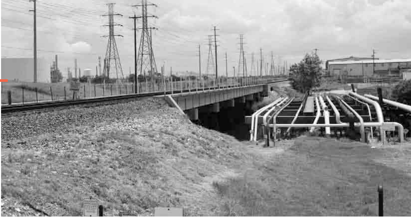
PASADENA BUFFALO BAYOU TRIBUTARY.
